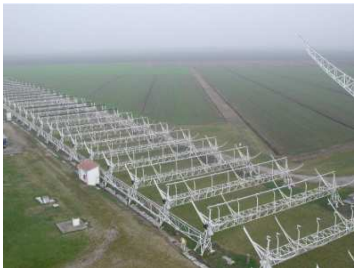
Fig. 4. Northern Cross North-South branch (credit: Fabbri Pietro)
